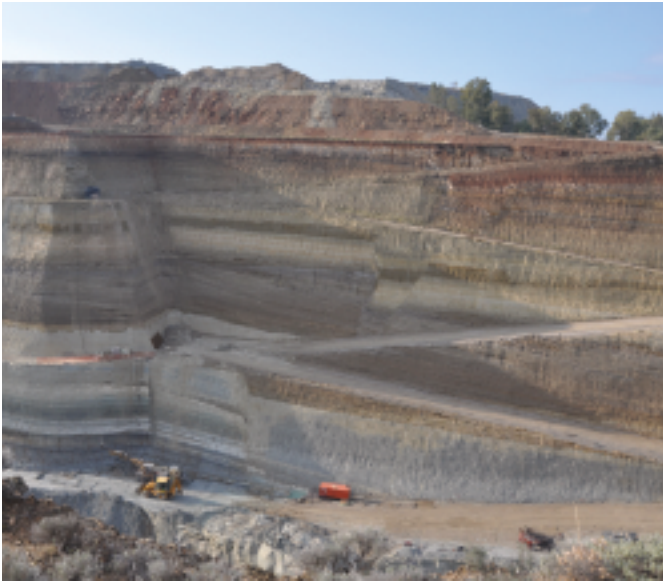
Normal faulting in the Corinth Canal, Greece
